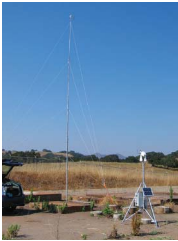
RSR system with 10 meter wind measurement pole installed for PV system site evaluation in California
